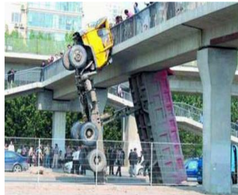
Figure 2. Dump truck-bridge collision
