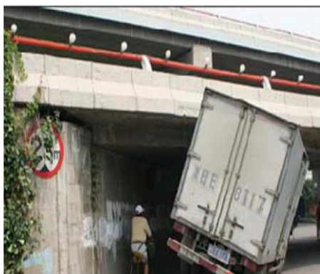
Figure 1. Cabin vehicle-bridge collision
