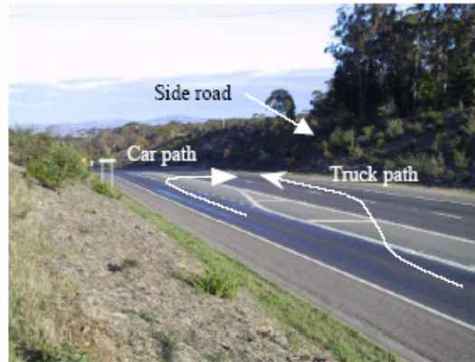
Photo 3: Crash site inspection
